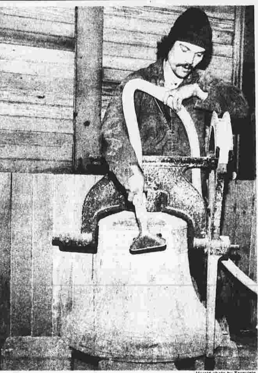
David Coon of Manchester vacuums the copper bell that until recently hung in the tower of the Clocktower Mill. The bell is now in the former chapel of the Cheney Bros. mill, which is being converted to 185 apartments. Coon works for the contractor on the conversion.
